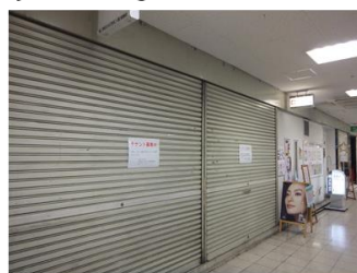
Deterioration of facilities around (low conviviality)
